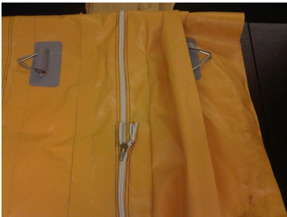
PVC overlapping on the outside of the Duct. Keep the Zip free from dirt.
